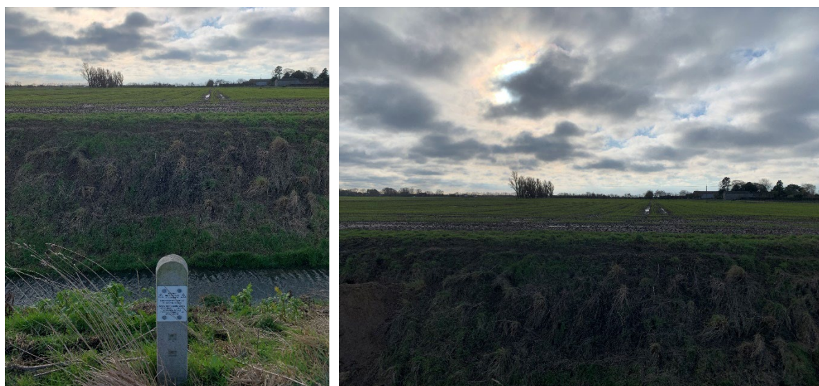
Photos 22 and 23: Nearby Buried Cables
